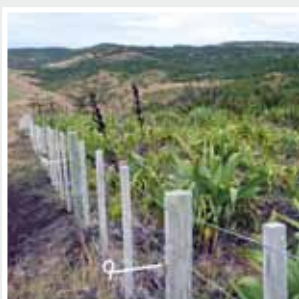
Electric outrigger used to protect fences from being pushed over by cattle. Image taken on Pitt Island. Photo by Amanda Baird.
